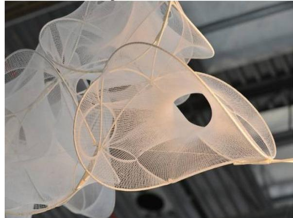
Figure 14. Calibration of flexible textiles to enable the structure of a surface of 27sqm. Calibration of these physical and morphological parameters allow the model to rely solely on a fixed two points (on the floor, a large entrance between the front and rear gallery spaces) to create a state of balance.
