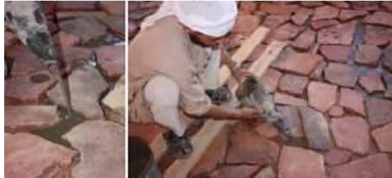
Pic.(15) rock flooring
