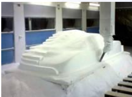
Milling the mold from blocks of lightweight polystyrene (Styrofoam) using milling CNC machine.
