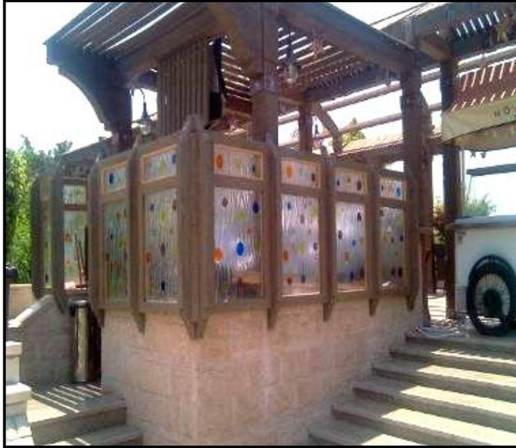
Figure (13) shows a kiln formed glass partition
