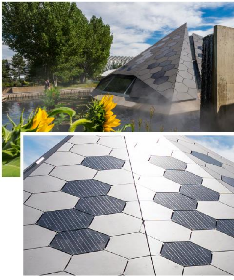
Figure (23) The Science pyramid, in Denver Botanic Garden, the designer has integrated hexagonal crystalline silicon photovoltaic glass modules with a custom-made design
