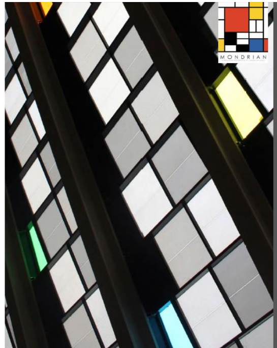
Figure (25) Refurbishment of the Historic food market of Bajer (Spain). Installations of 175m 2 photovoltaic skylight, with different degrees of transparency and colours form a mosaic inspired from Piet Mondrian, part of the power generated is sent to be stored in batteries, and the rest is sent to the grid for the building's own consumption.
