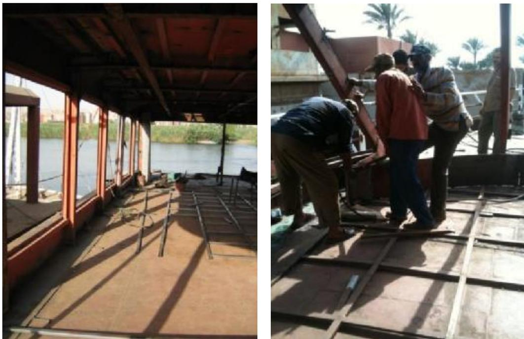
Picture (6) iron structure on the floor is divided according to the measurements of the Acrylic tiles
