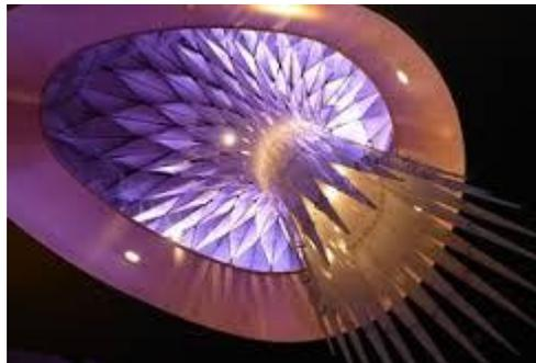
Picture (5) Acrylic used in cladding the ceiling
