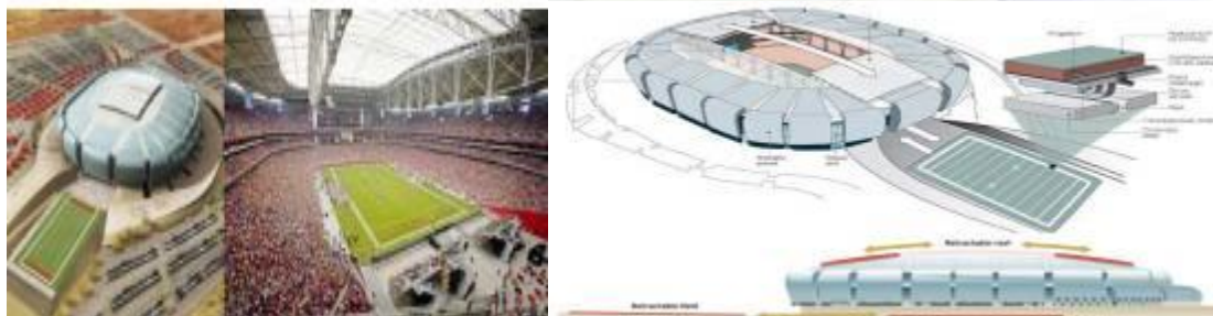
Fig (4) University of Phoenix Stadium is open from the inside and from the outside and the roof and the roof is closed - and Aksnumtry interface illustrate the movement of the roof (Iron + PTFE material transparent half) and pitch (Iron + polymers like substance Genotextile fabric + concrete and tin Marj) in Phoenix Stadium
