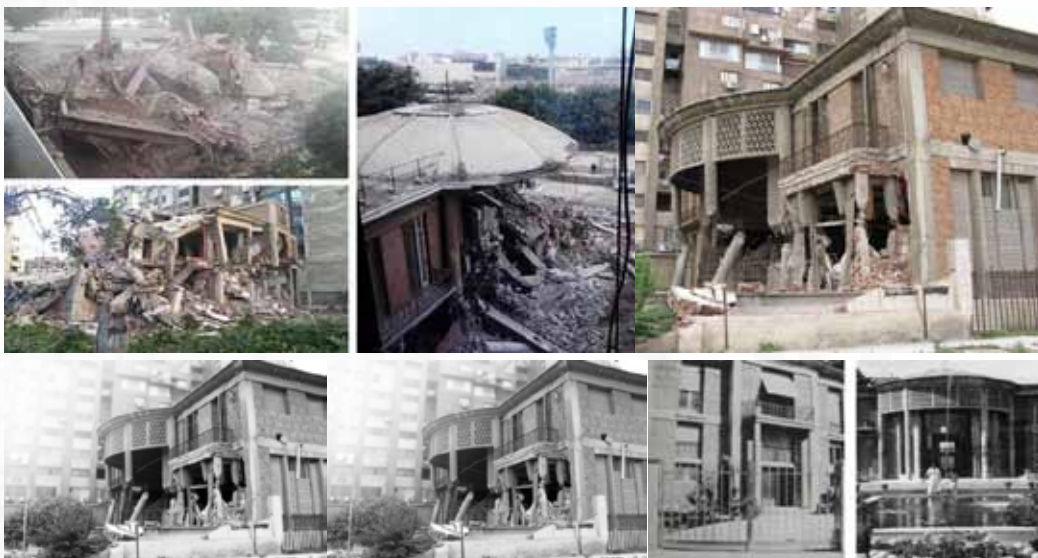
Figure 3. villa Aghion design after the collapse in Alexandria.
