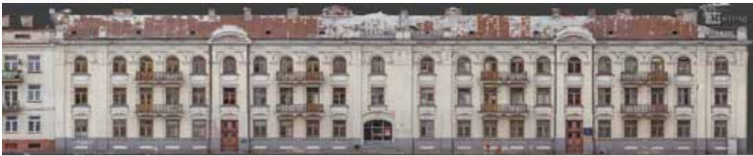
Figure 56. Historic Elevation in Plock in Plock, Poland (“Historic Elevation in Plock,” 2018).
